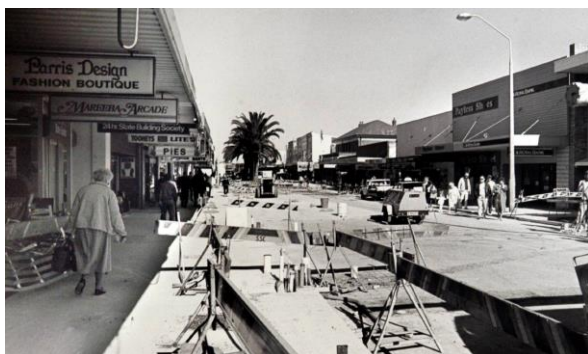
Figure 10: The plaza under construction in 1988 (source: Council)
