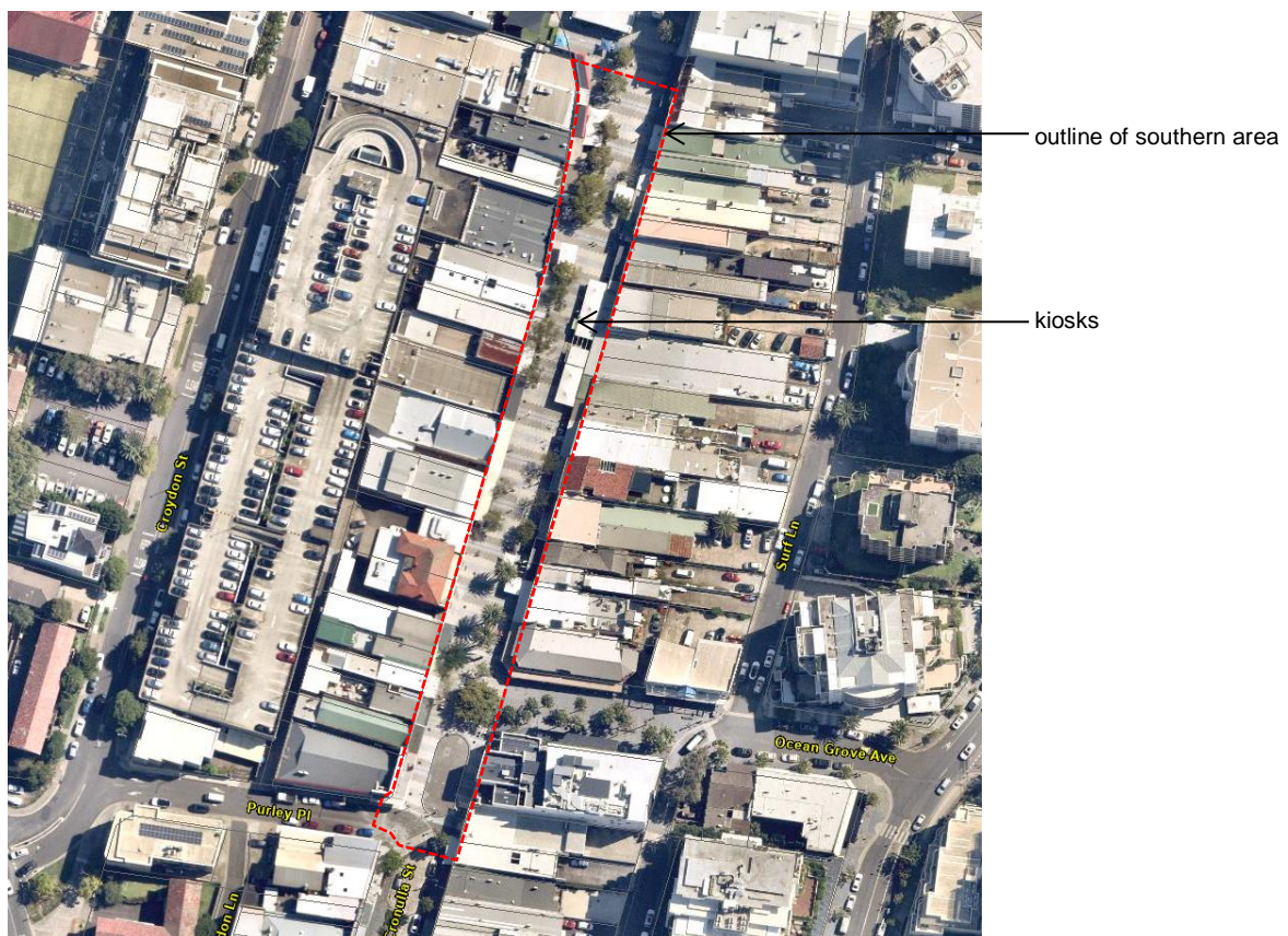
Figure 20: Southern area of the plaza (source: Council)
