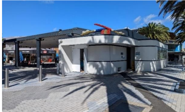
Figure 14: Toilet building and canopy over stage and seating (source: Council)
