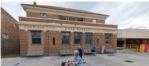
Figure 51: Cronulla Post Office (local heritage item) (source: Google)
