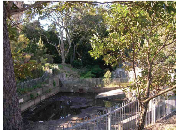
Photo 2 – Gwawley Creek & GPT downstream of Box Road
