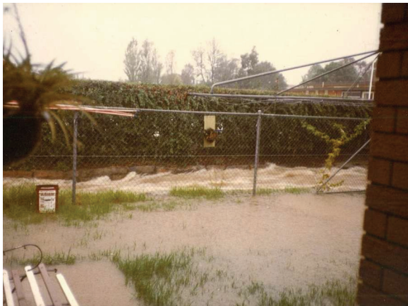
Photo 5 – Stormwater channel, Dyinda Pl, Miranda (1983)
