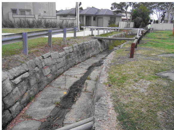
Photo 3 – Open Drain in Southern Subcatchment
