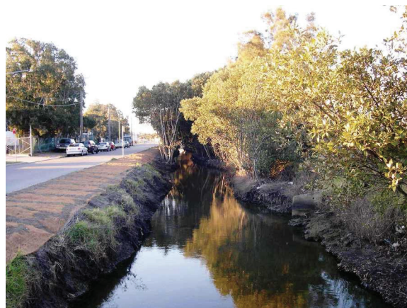
Photo 4 – Production Rd Channel downstream of Bay Rd
