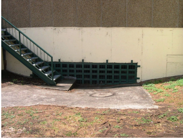
Photo 11 – Inlet to main culvert under Southgate (Oct 2007)
