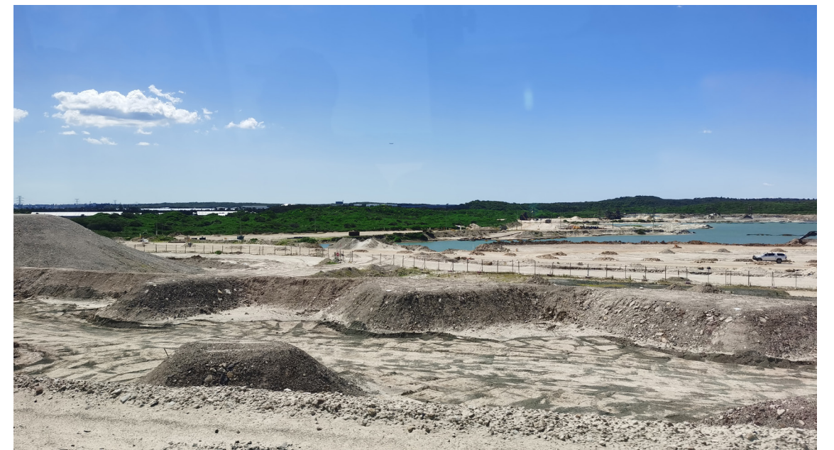
4. Altered landform with sands extraction and storing on site
