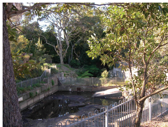
Photo 2 – Gross pollutant trap downstream of Box Road
