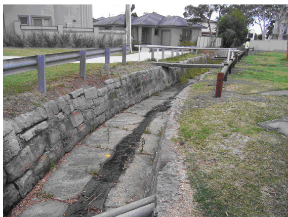
Photo 3 – Open drain upstream of Port Hacking Road
