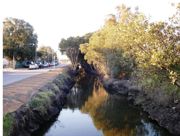
Photo 4 – Production Road Channel
