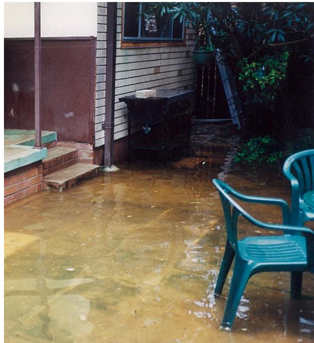
Photograph 2: Flooding at 87 Torres Street during the May 2003 storm
