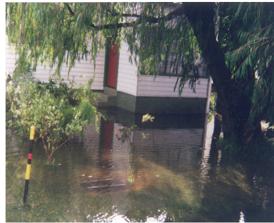
Photograph B10: Flooding outside 61 Tasman Street
