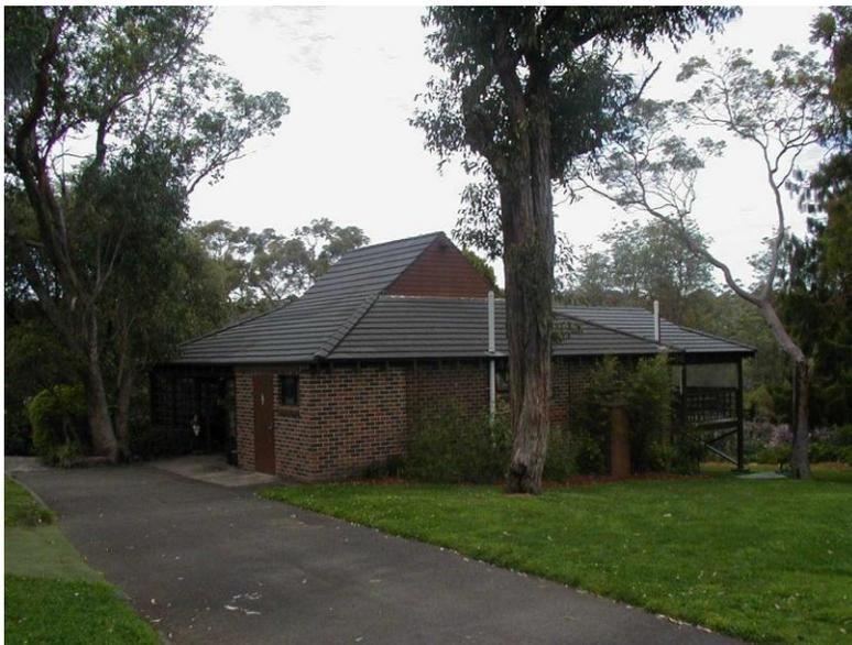
The teahouse is of timber frame construction with brick veneer exterior cladding on the western and part of the northern wall. The balance of the external walls are of timber framed glass. Timber framed sliding glass doors provide access from the main gardens to the tea rooms. A second entrance is accessed from the north. The roof cover is of concrete tiles.
