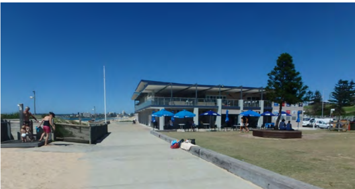
Wanda SLSC eastern frontage
