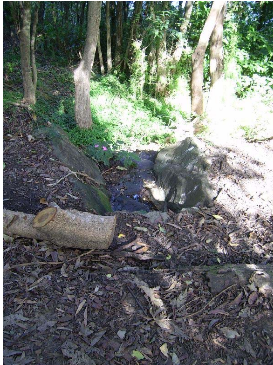
Figure 7.17 Stone culvert running under track
