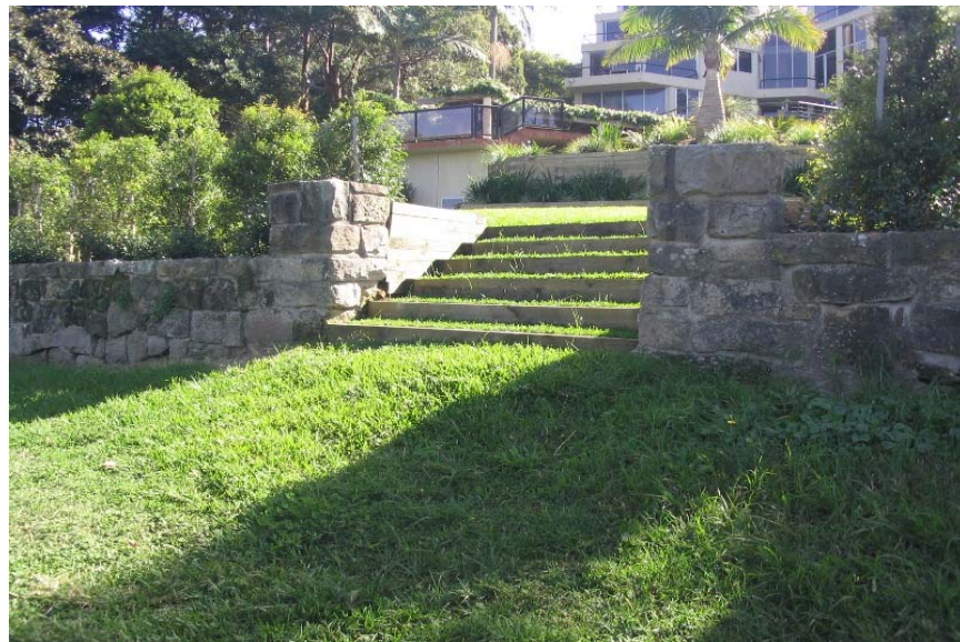
Figure 7.4 Sandstone boundary wall at 82 Lilli Pilli Point Road.
