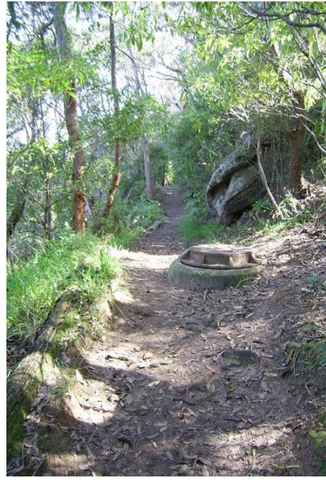
Figure 7.16 Track facing south west with raised sewer line access hatch
