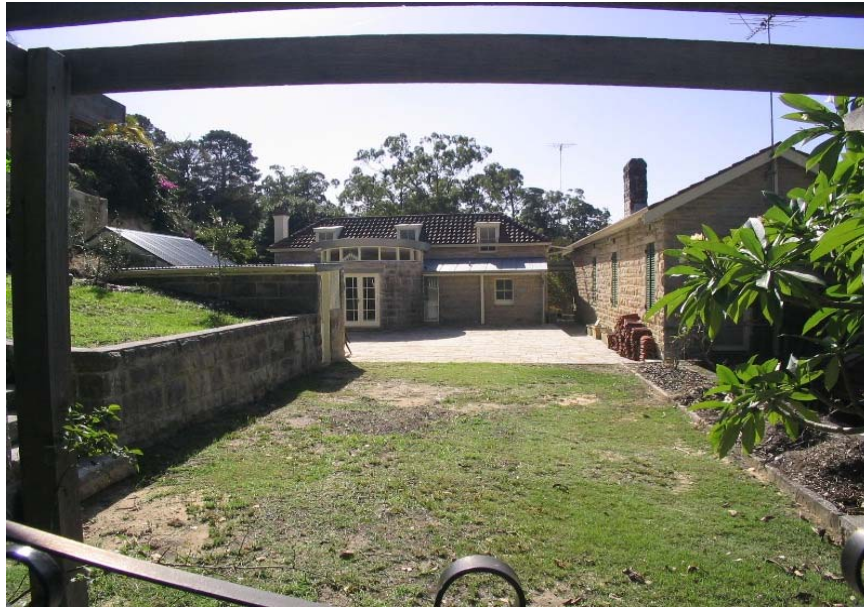
Figure 7.3 Looking north to the rear of Nuimburra showing three construction phases.
