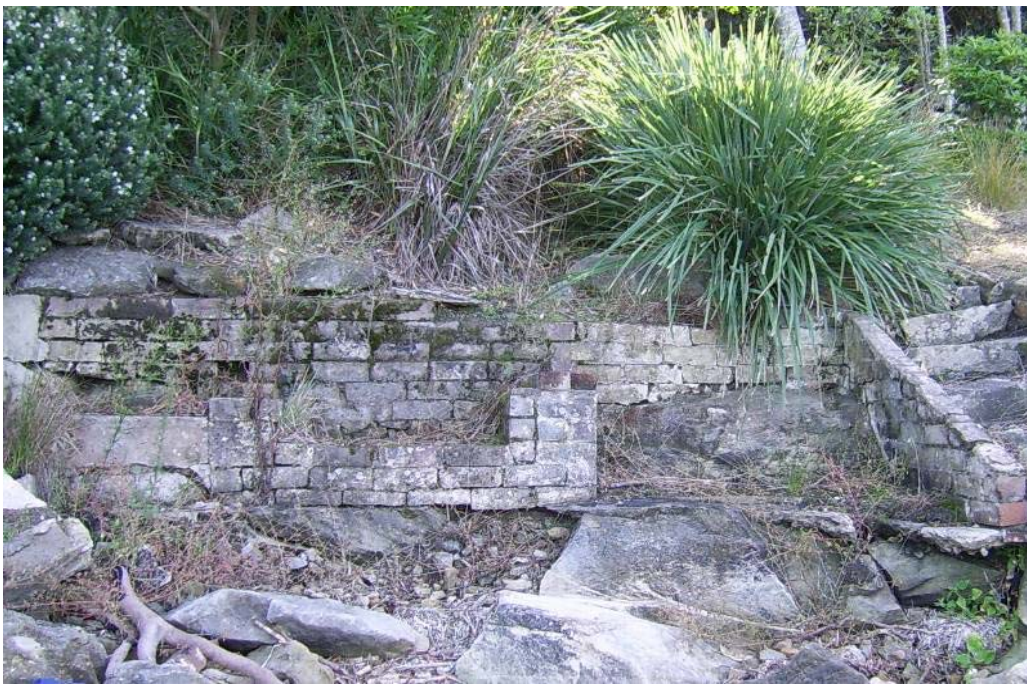
Figure 7.13 Remains of a brick chimney base from a demolished building associated with PO 35.
