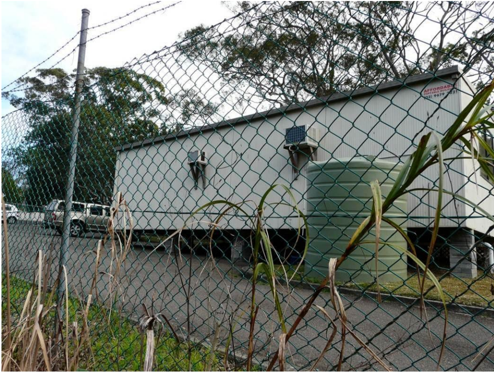
Figure 3: Faecal drop on demountable building within the school
