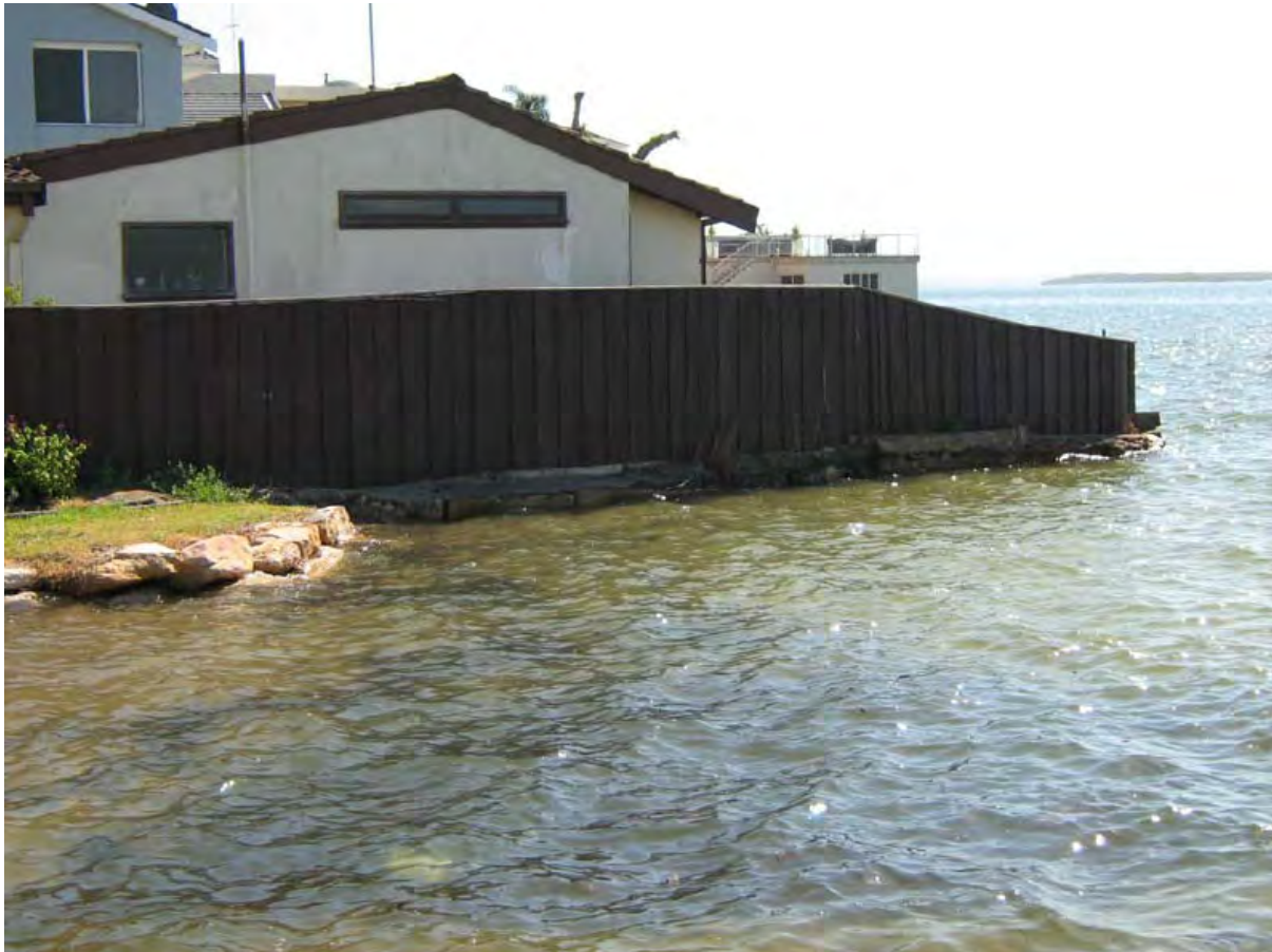
FIGURE 5.2 – King Tide at 64 Woodlands Road, 9.46 a.m., Monday 12 th January 2009 (Source: Council)
