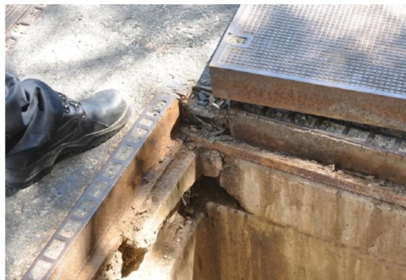
Photo 8 - Structural Defects around Frame
