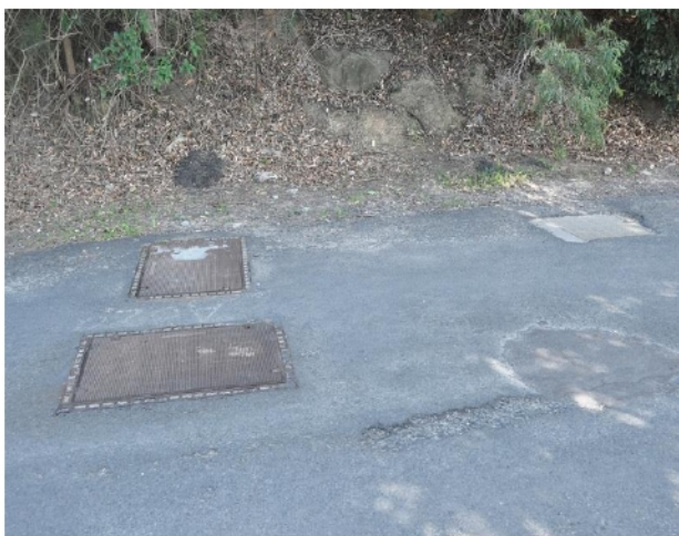
Photo 5 - Humegard™ and Junction Pit AB2
