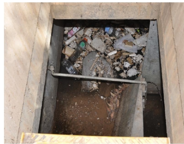
Photo 6 - Litter & Boom inside Humegard™
