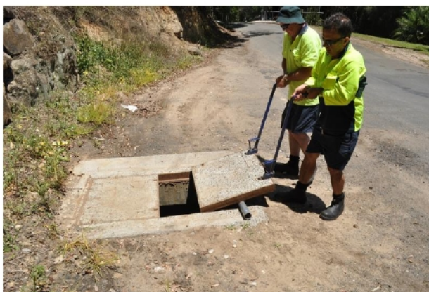
Photo 3 - Removing the Lid from Pit AG5
