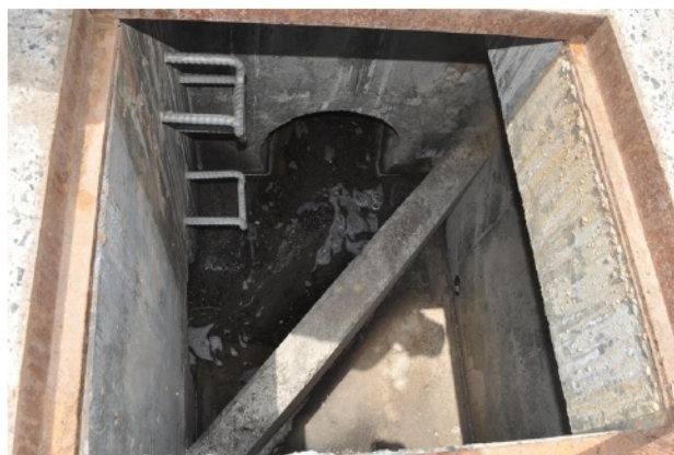
Photo 4 - Debris & Sediment within Pit AG5
