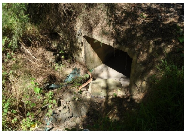
Photo 12 - Inlet to Existing Box Culvert
