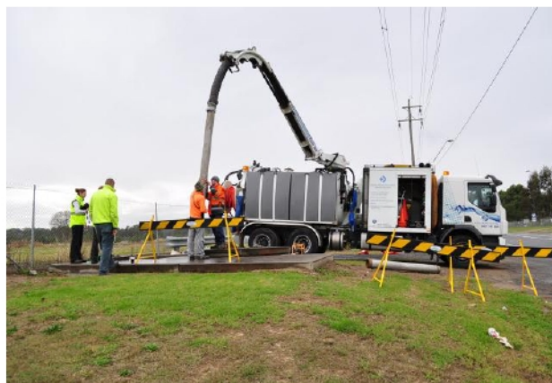
Photo 2 - Cleaning an Underground GPT
