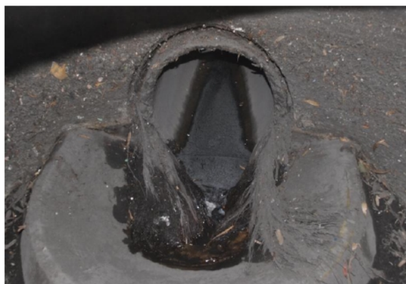
Photo 10 - Inlet Blocked by Tree Roots
