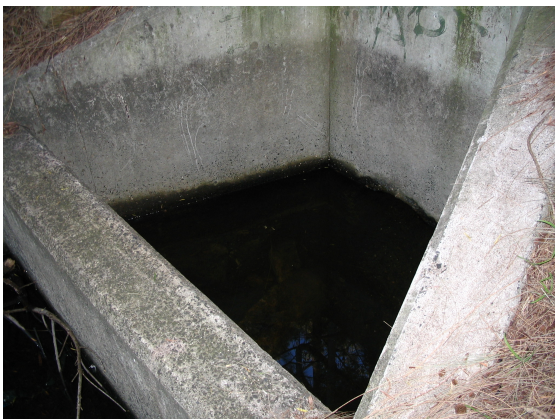
Figure 7: Inlet Structure to Wetland with Surface Skimmer and Energy Dissipation Baffle.
