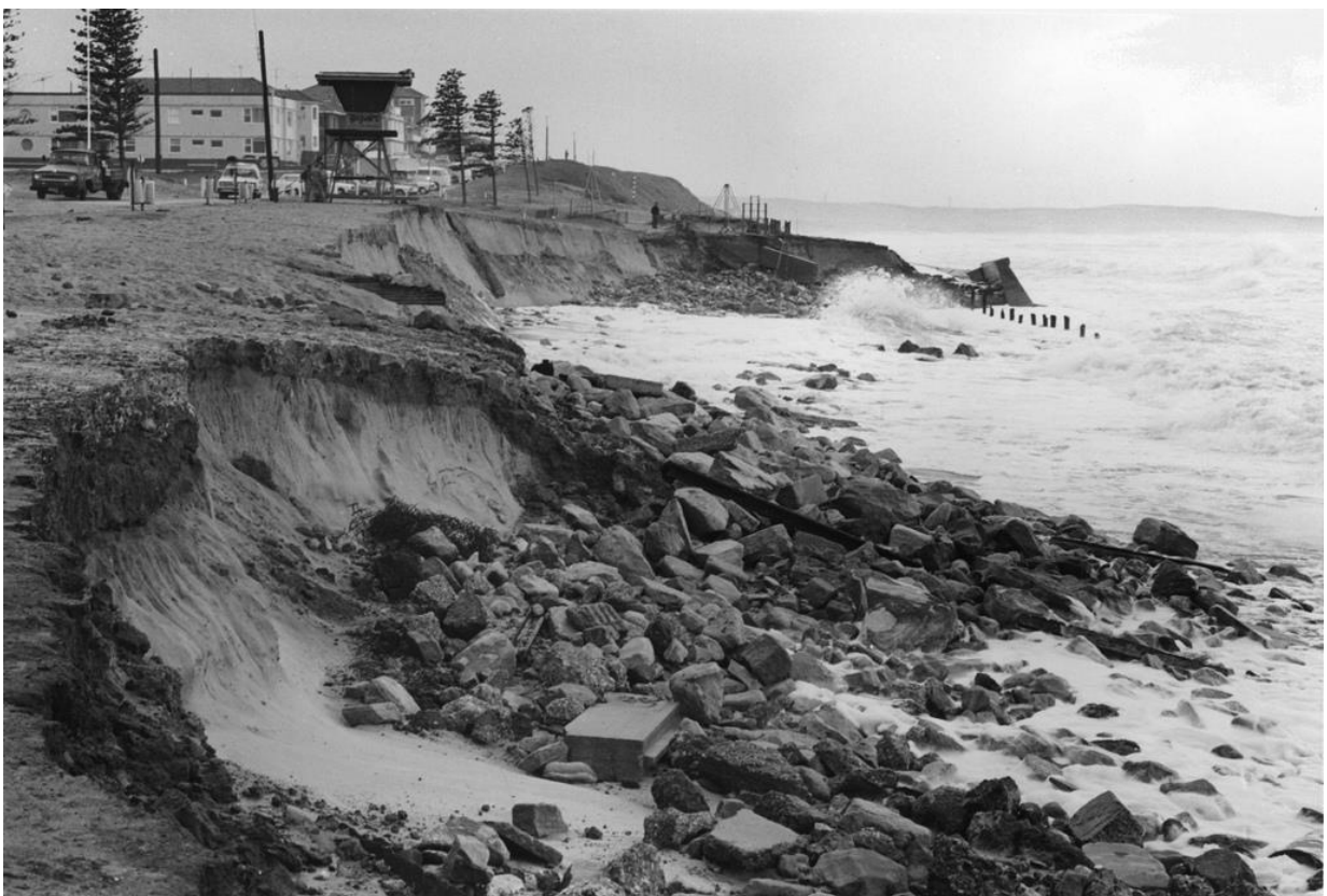
Figure 8-13: 1974 Storm Erosion at North Cronulla Beach
