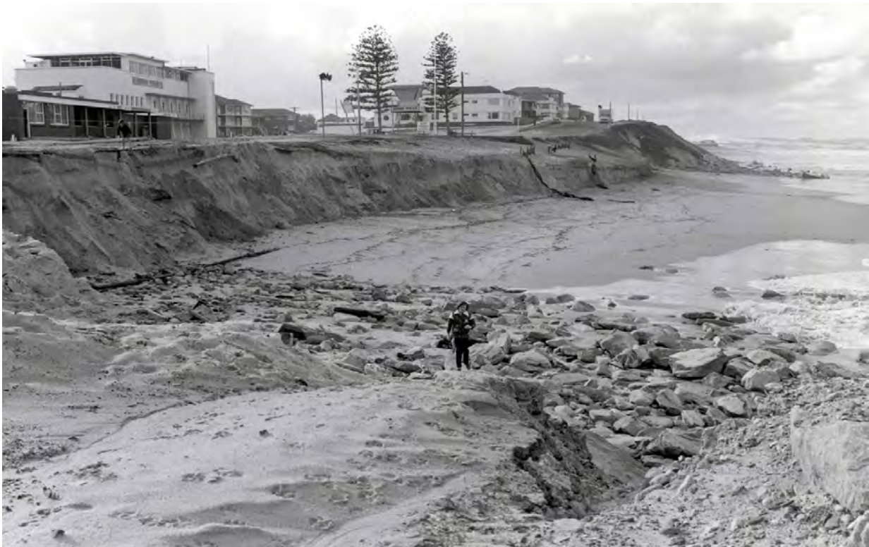
Figure 8-12: 1974 Storm Erosion at Dunningham Park
