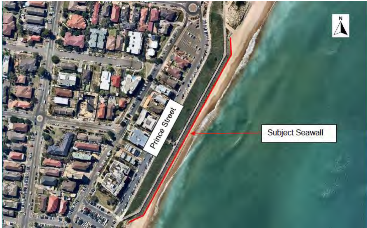
Figure 8-8: Prince Street Seawall
