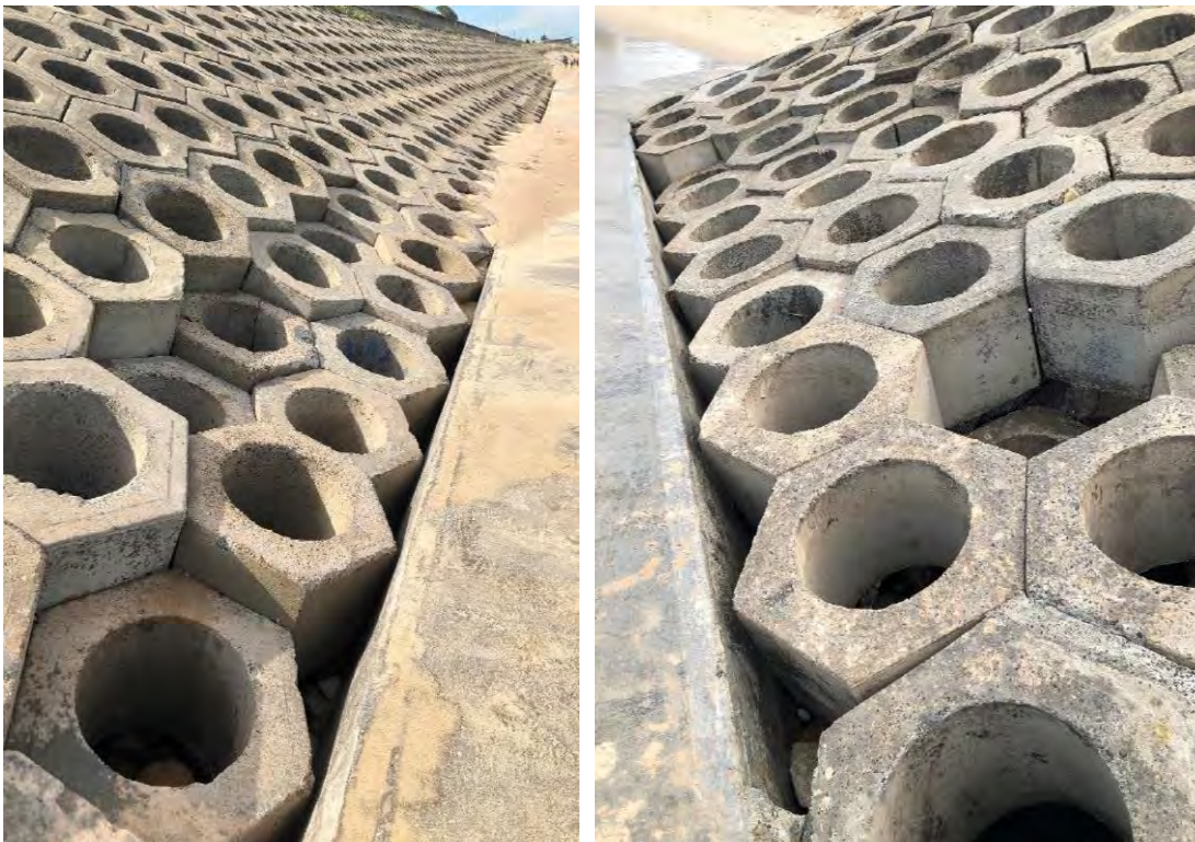
Figure 8-10: Subsided Seabee units (left) and Seabee units spanning over large cavities where individual units have dropped (right)
