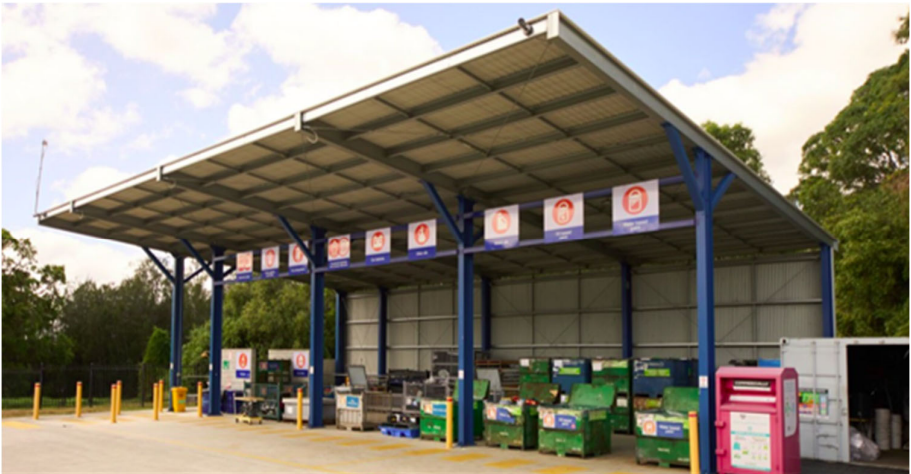
Figure 18 An example of a Community Recycling Centre (Campbelltown)
