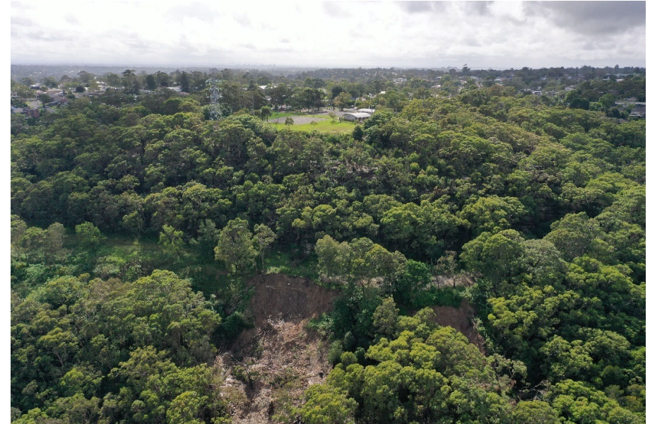
Figure 12 Ferntree Reserve Landslip Aerial
