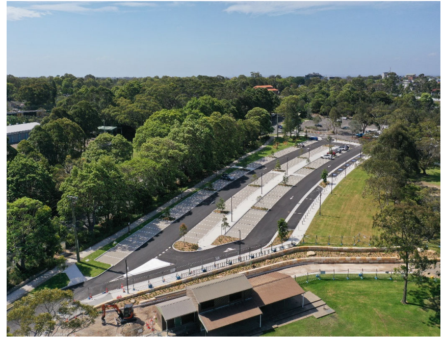
Figure 20 Waratah Park Car Park
