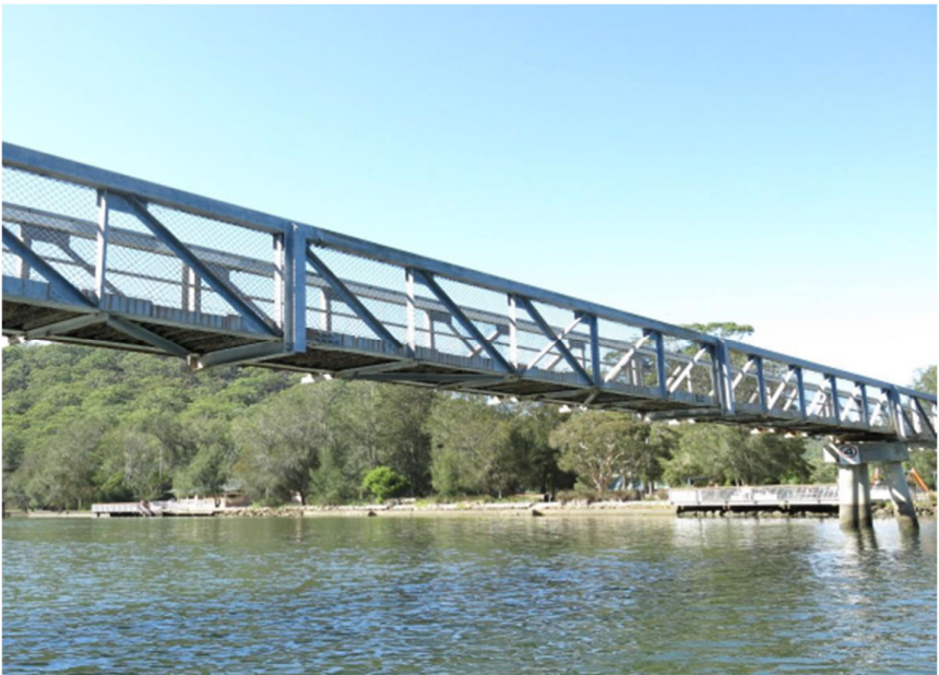
Figure 15 Existing Prince Edward Park Road Pedestrian Bridge
