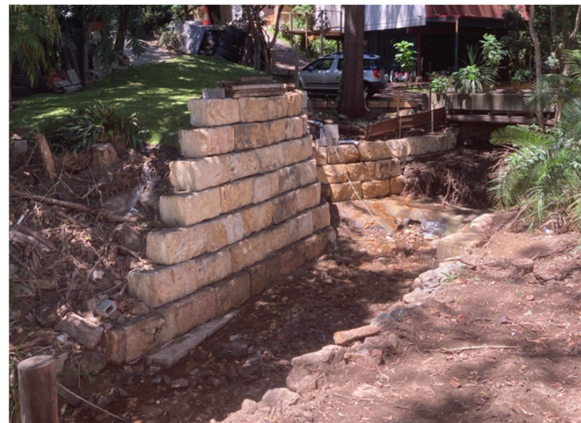
Figure 36 Open Channel Restoration at Old Ferry Road, Illawong
