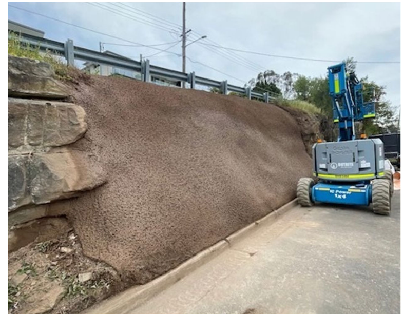
Figure 23 Embankment Stabilisation – Attunga Road, Yowie Bay
