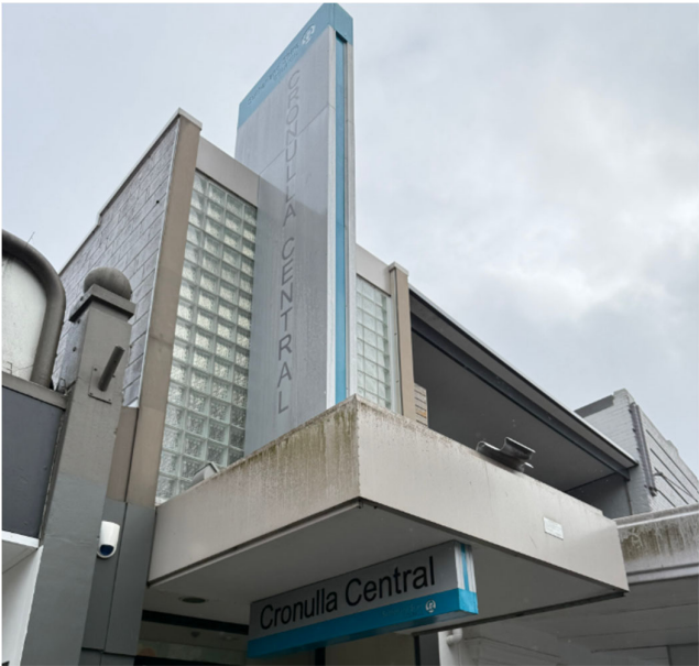
Figure 5 Existing Cronulla Central Façade (Town Centre entry)
