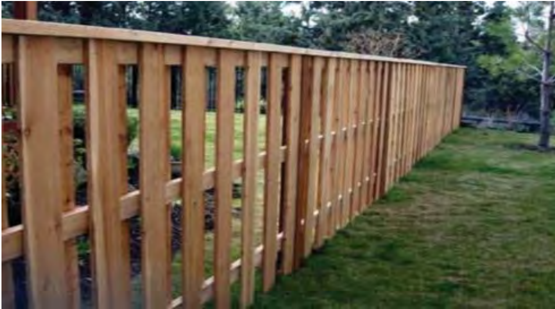
Figure 11: Example of a timber paling flood fence
