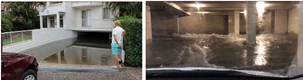
Photo 10: Inundated Basement Car Parks
