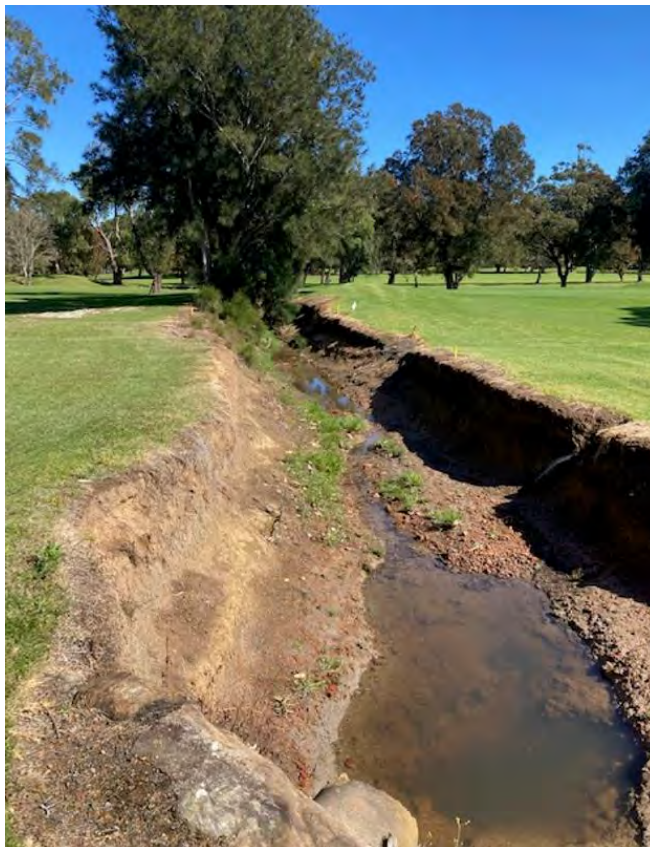
Photo 12: Channel from under Woolooware Road into golf course cleared of vegetation
