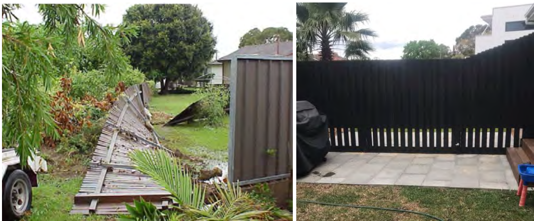
Photo 9: Fences Damaged in a Flood and Flood Compatible Fencing
